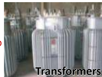
Examples of Devices Containing PCBs
