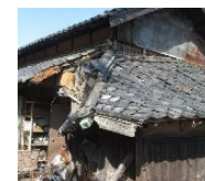
A collapsing roof requiring emergency substitute enforcement
