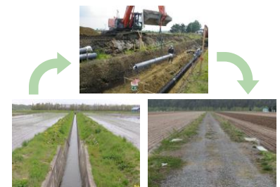
Converting open irrigation channels into pipelines and widening farm roads
